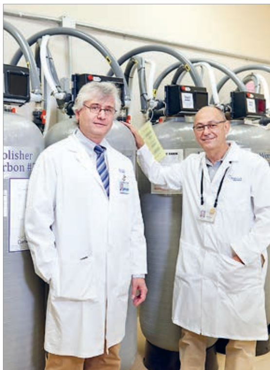
Ira Meisels, MD, left, and Robert Levin, Director of Biomedical Services for the Renal Research Institute, at the Avantus Upper Manhattan Dialysis Center. The tanks behind them, where sodium bicarbonate powder is mixed with water, may soon be replaced by disposable bags that greatly reduce the risk of contamination.
